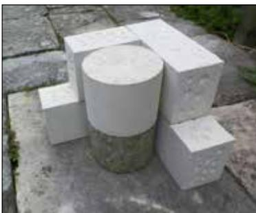
*The two courses of the Nook Shaft display, showing the positioning of the new shaft stone alongside the rectangular blocks of ashlar and the original whistle stone*
