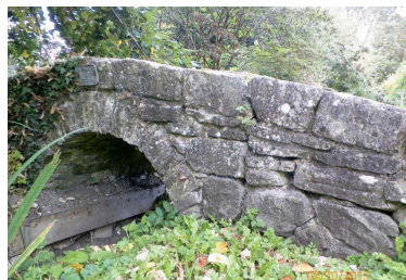
Stone bridge across the stream running through the garden of Silverstream, built from the ashlar stones found in the garden rockery.
