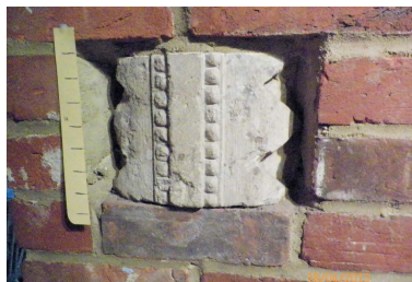
12th century Romanesque billet moulding stone which was found in the garden of Silverstream, Headbourne Worthy. It was later reused as a feature in a brick chimney in an extension to the cottage. The stone was originally part of the stone chimney in the cottage.
