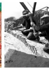
Men using sledgeshammers to bang in wedges to split stone
