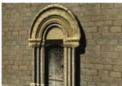
The digital image of the doorway showing the voussoir forming part of the arch.
