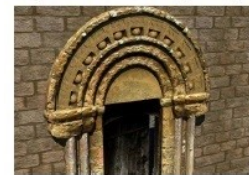
The digital image of the doorway showing the springer stone at the conclusion of the arch.
