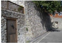
The west wall adjoining Hyde Gate looking north
