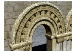
The digital image of the doorway showing the decorative voussoir forming part of the arch
